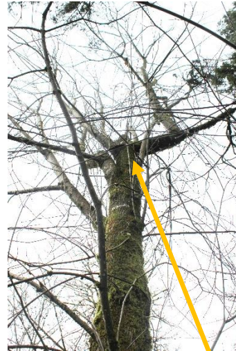
7706 Bigleaf maple, previous top loss, dead wood, carpenter ants
