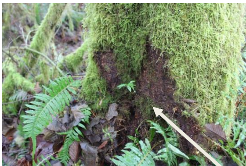
8225 Red alder: decay at root crown, carpenter ants
