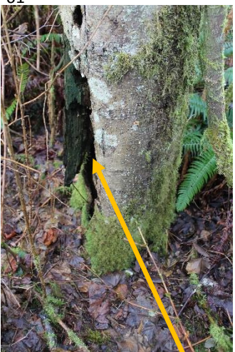
7416 Red alder: decay @ root crown
