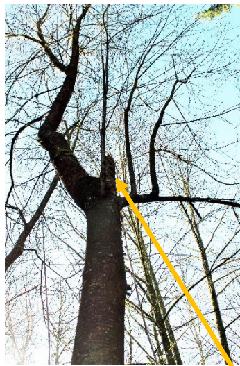
7589 Cherry: Co-dom failure, decay throughout
