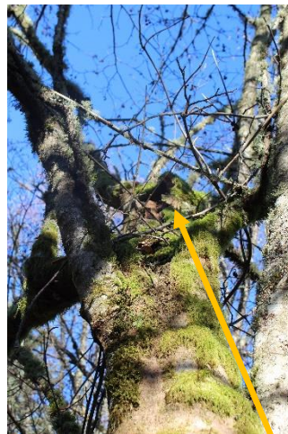
7579 Red alder: previous failure of a large portion of top, decay throughout
